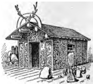
Mineral Cabin, New Mexico.
